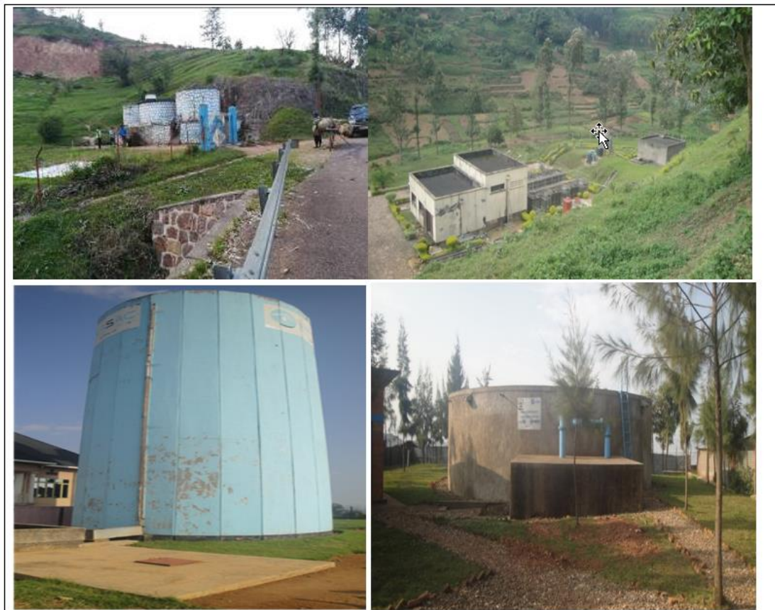
Plate 1 showing the Water Tanks to be rehabilitated in this project
