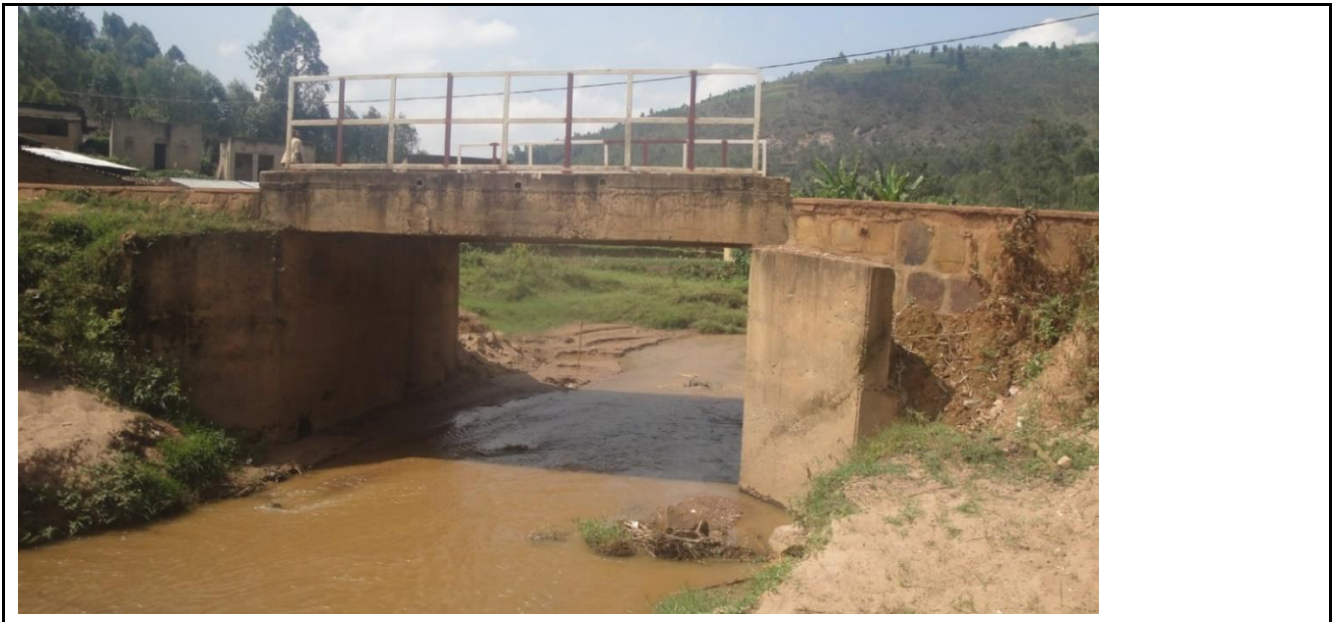
Figure21: A Bridge on One of the Roads in Gicumbi Town
