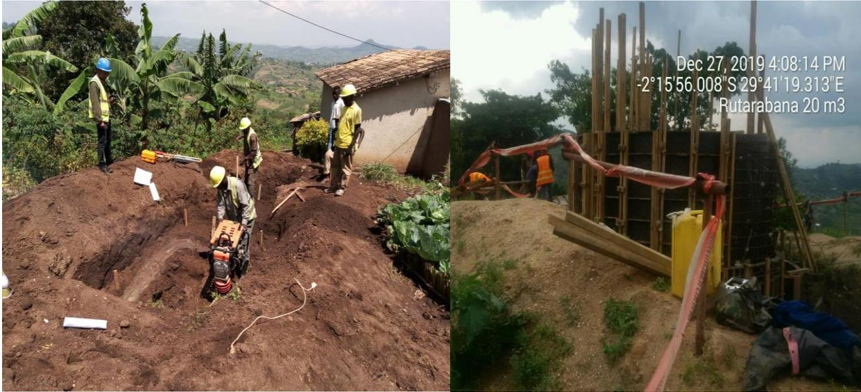
Picture 1 [above] shows excavation on a site to be constructed a water kiosk in **Ruhango** and picture2 is about fixing formworks on **Rutarabana (Gitwe) 20m<sup>3</sup>** reservoir.
