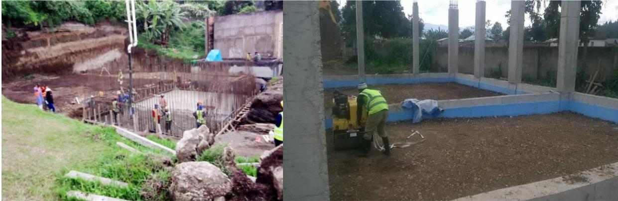
*The raft foundation concrete casting for the valve room of 2500m<sup>3</sup> RWAZA reservoir are complete and the shear walls re-bars installation are ongoing. Photo 2 is the backfilling and compaction of chlorine and Chemical building.*
