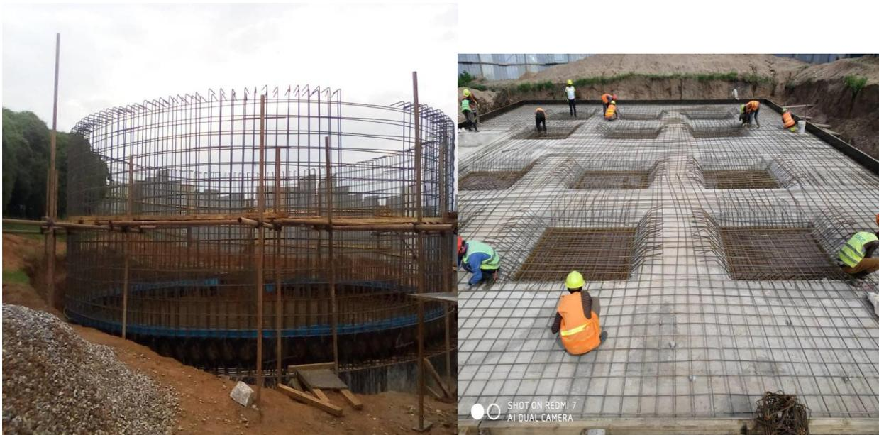
Picture 1 [above] shows steel works at **Gihuma WTP 200m<sup>3</sup>** reservoir and picture 2
