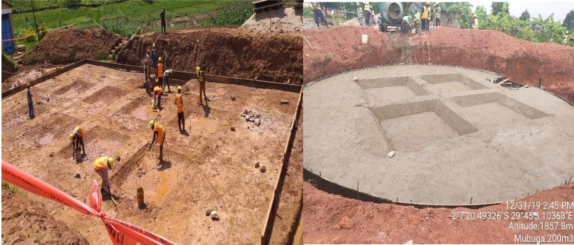
Picture 1: [above] Rebate fixing at a bottom slab of **Mpanga 500m<sup>3</sup>** Reservoir and
