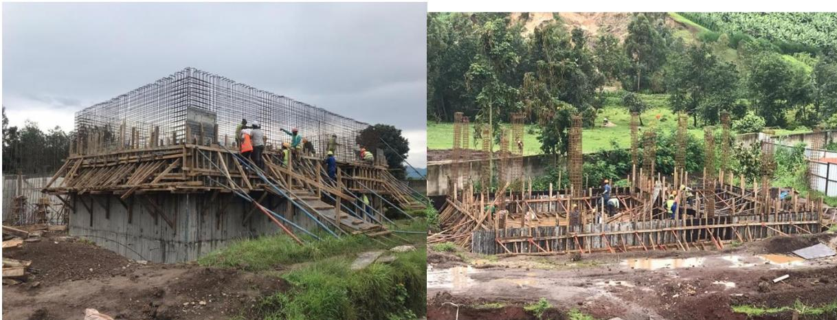
*Picture1: 6000m<sup>3</sup> reservoir valve room ready for the second casting while the shear walls of 1.8m for the chemical Chlorine building was ready for casting as shown by picture#2*
