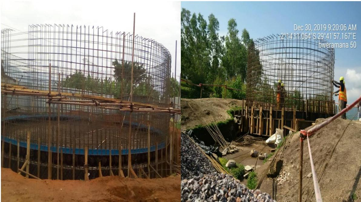
Picture 1[above] shows steel works on the structure of **Muhanga Industrial park 400m<sup>3</sup>** reservoir and picture 2 shows the steel works on the structure of **Bweramana 50m<sup>3</sup>** reservoir
