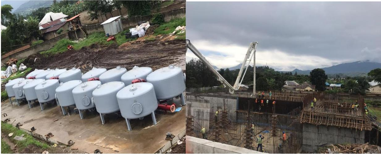
*The Omni Filter System (OFSY) filters are already installed in their positions (picture1) and concrete casting works for the left side shear walls of the 6000m<sup>3</sup> Reservoir and its valve room (picture 2)*
