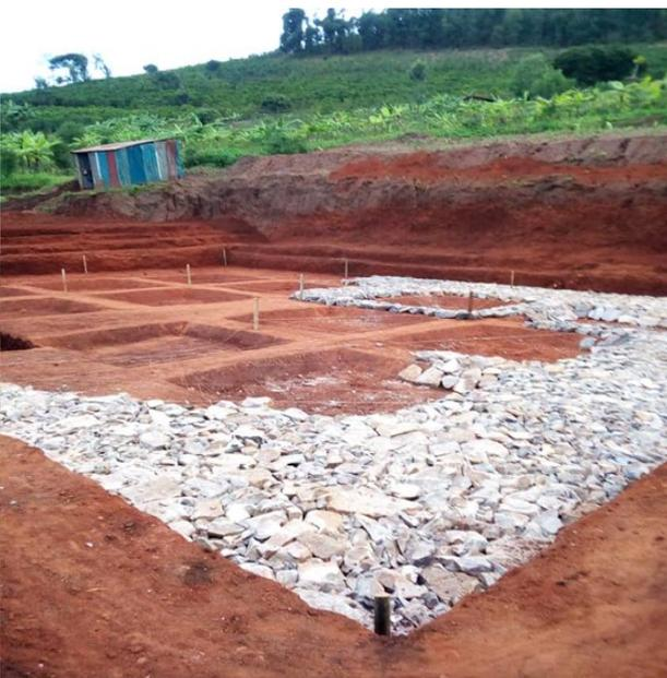
*Picture 1 and 2 show site camp installation, photo3 shows Clearing, Excavation, levelling, setting out, DCP, access road for Kanazi 2000m<sup>3</sup> reservoir location while picture number 4 shows hard core laying at 1000m<sup>3</sup> Sovu reservoir.*
