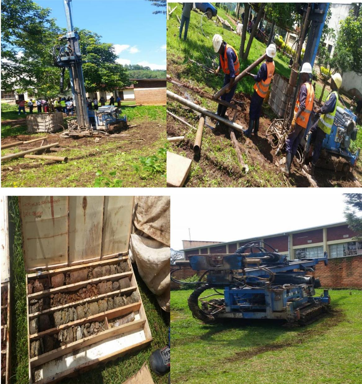
*Photos: Sampling the soil for testing their bearing capacity.*
