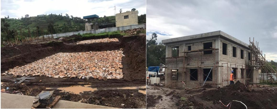
*Picture 1: The excavation works for the clarifier and sedimentation are completed.*
